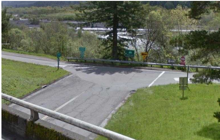
Figure 23 A Potential Stop Location on Glendale Drive's Off-ramp
